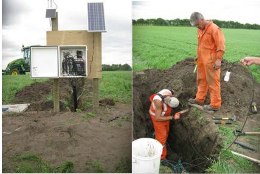
Figure 7. Site installation for AAFC in situ soil moisture sites.
